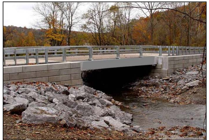
Figure 6. Elevation of the modular Erie County NY bridge that was built in 30 days.
