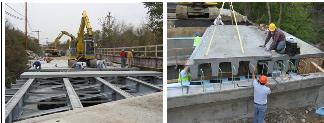
Figure 13. Composite Advantage 14 uses a 3D fabric and a special resin transfer molding process to fabricate both decks and superstructures.
