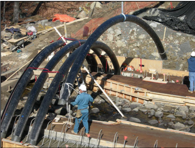
Figure 10. CFRP tubes filled with concrete constitute arches for a 34' bridge.
