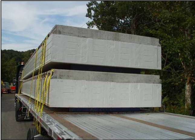
Figure 5. Two 25,000 lb. hybrid superstructure panels delivered by truck to the site.
