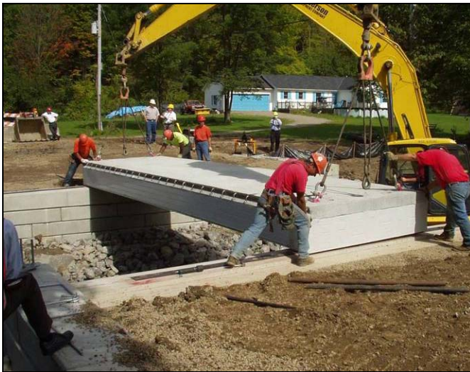
Figure 7. Backhoes were used to lift the superstructure panels into place.
